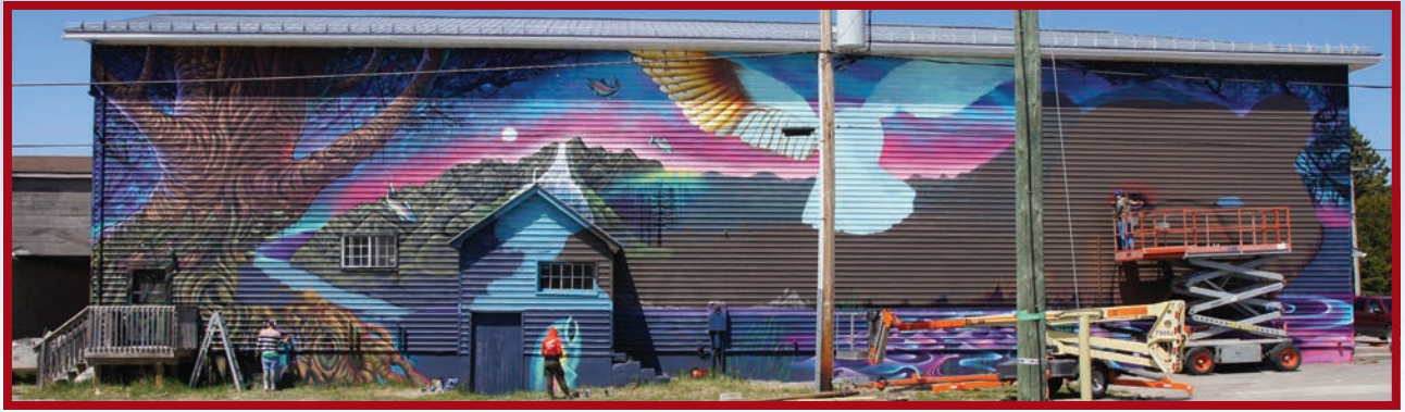
▲ Work in progress: in May the mural was being painted.
